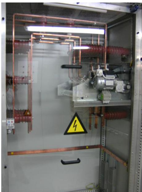
DC 2 IN + 1 OUT 7.2kV 630A 3p , inside view
