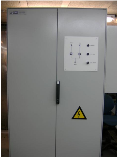
DC 2 IN + 1 OUT 7.2kV 630A 3p , outside view
